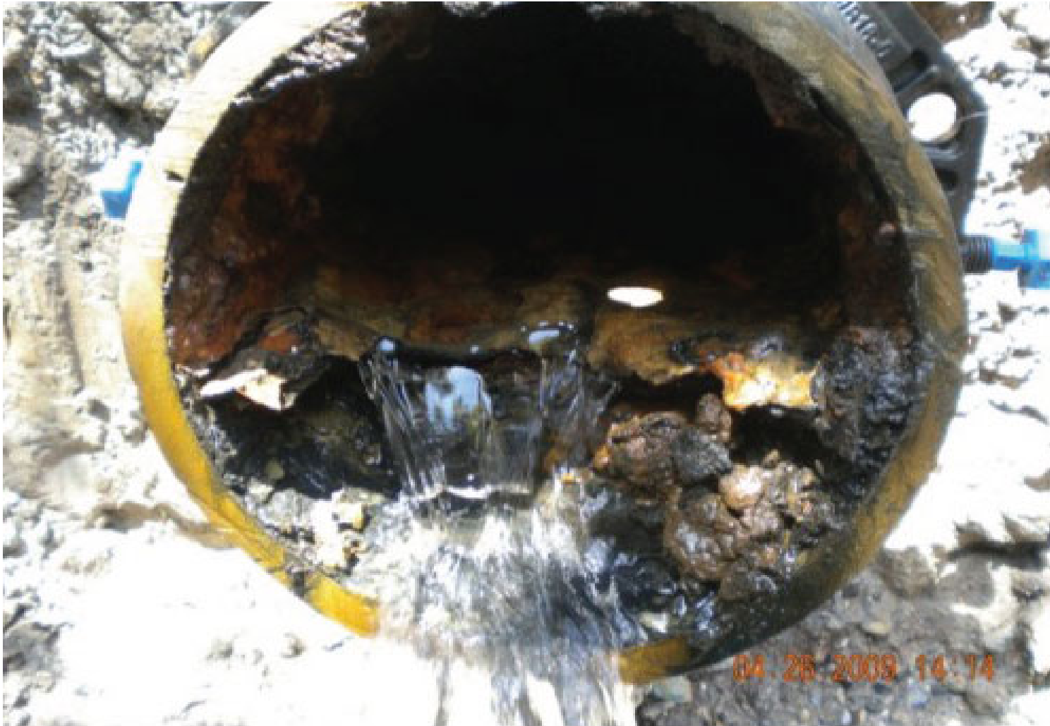
A 100 year old pipe in a metropolitan area
